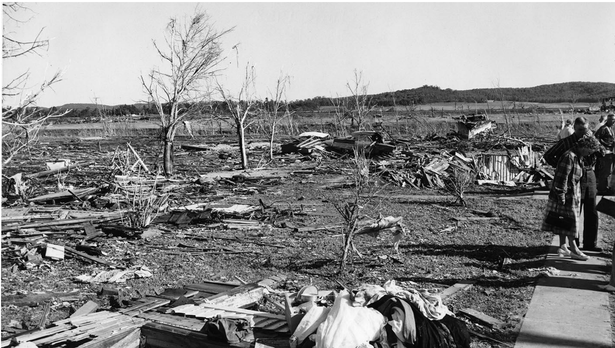
Residential area in Colfax destroyed by tornado, June 1958
