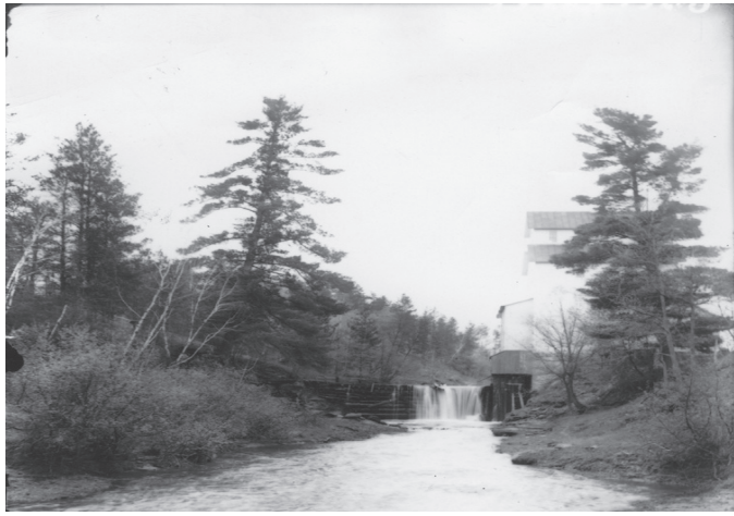
Looking upstream at Otter Creek Dam with part of mill showing
